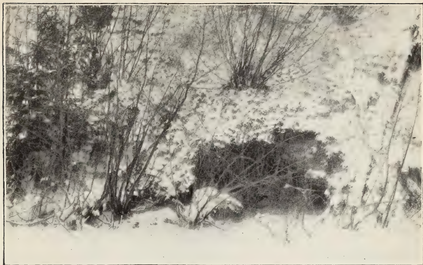
FIG. 1.—WASHING OF THE SHORE OF LITTLE TUPPER LAKE BY HIGH WATER, CAUSED BY AN UNNECESSARILY HIGH DAM.
